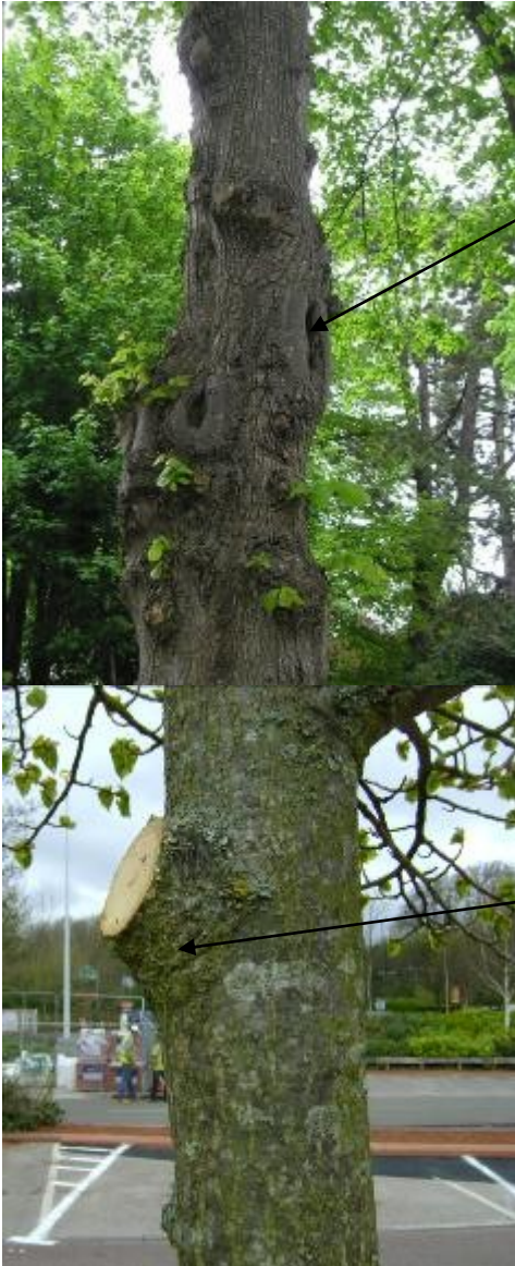
Flush cut that has led to decay in a Lime.
